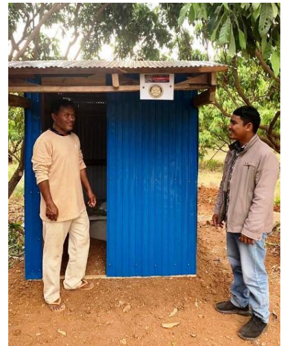
Latrine complete built
