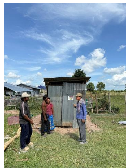
Latrine complete built
