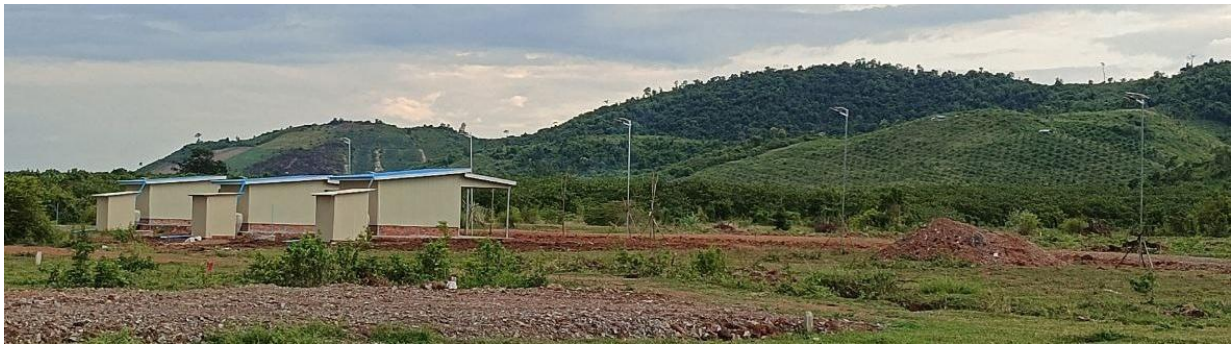
(Three house building in CFS village)
