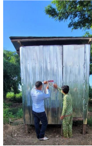
Latrine complete built
