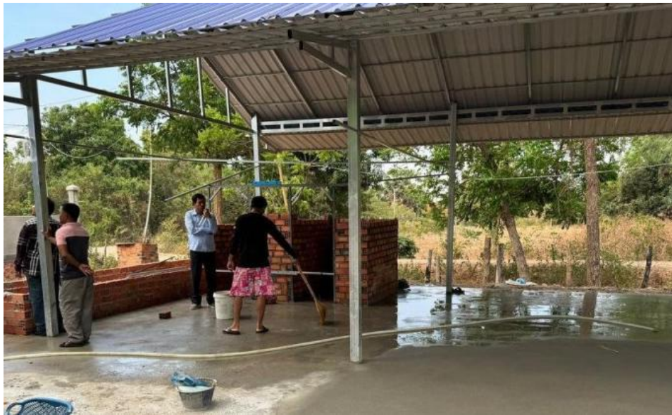
(Dr. Samnang director of CFS visited building progress)
