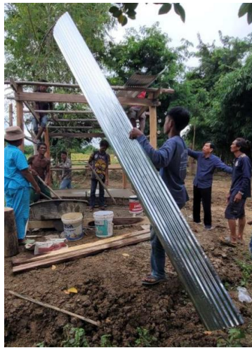
Helping each other to build
