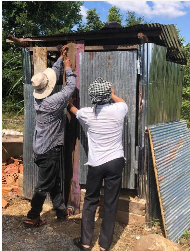
(We helped her to build a latrine)
